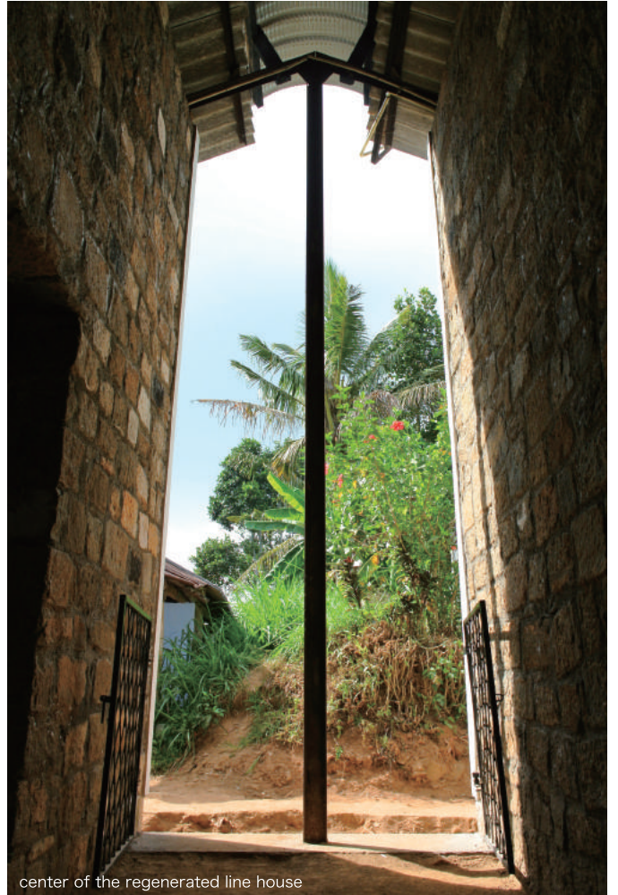
steel pillar which have supported the line house for 130 years and a boy, who is immigrant 5th
