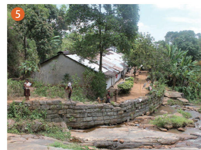
Existing line house There are 12 line houses where Tamil people have been living for more than 130 years since tea plantation was introduced here. They tell you that there used to be tea plantation in Bawlana.
