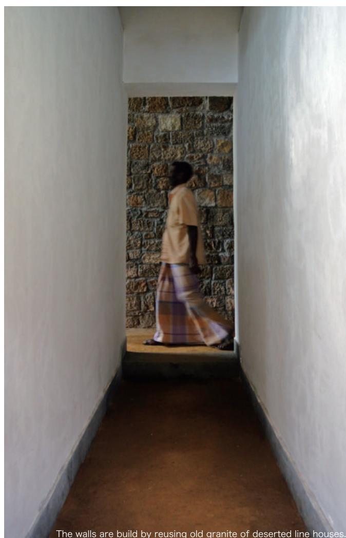
The walls are build by reusing old granite of deserted line houses.
